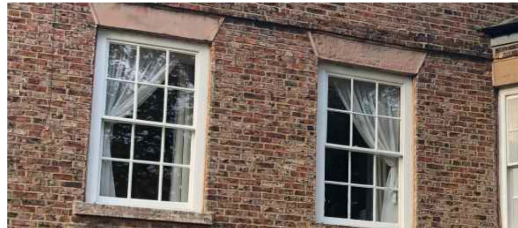
ORIGINAL SASH WINDOWS
